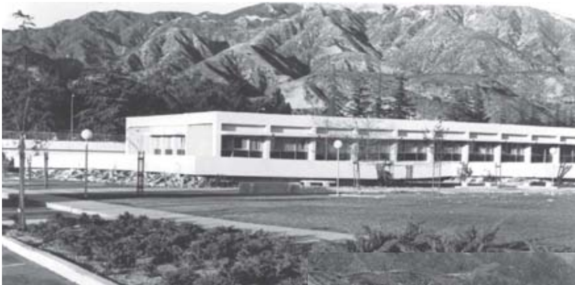
After the Earthquake
