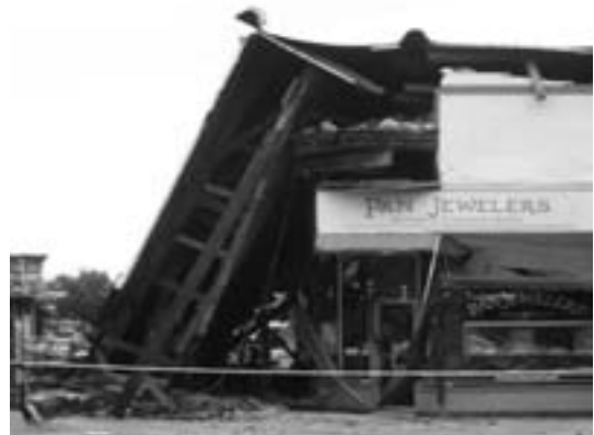
Figure 6 - San Simeon Earthquake, Dec. 22, 2003. The Acorn Clock Tower Building constructed of unreinforced masonry collapsed killing two people.
