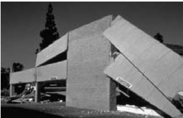
Figure 5 - Concrete Parking Structure Collapse.
